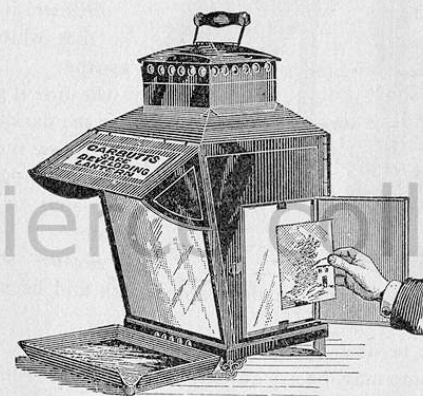
Lantern arranged for developing, and after fixing examining negatives by opal light.
